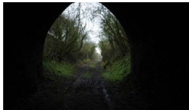
Old railway line on tunnel approach
