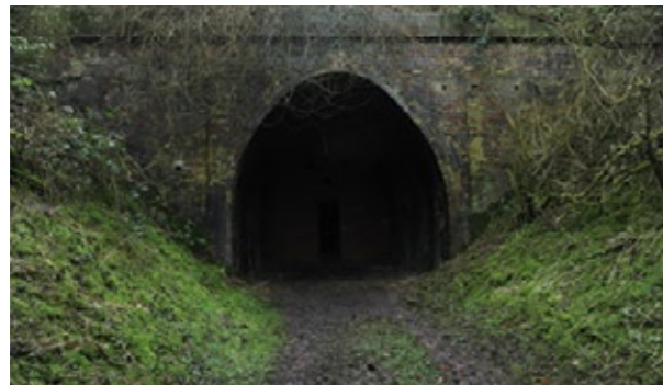
Withcall Tunnel entrance
