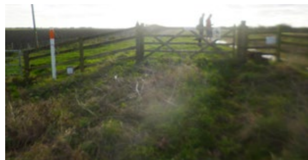
Canal access gates south of Bull Bank
